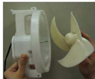
Separate a blade of a fan from a C-Fan motor shaft.
