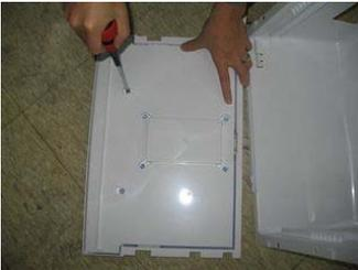
Loosen screws at bottom of a changing room cover.
