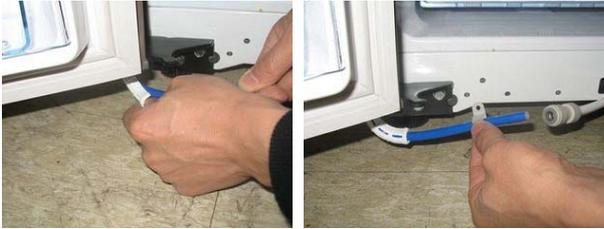
4 Fix connecting area between water supply hoses (fitting connection area) using screws.
