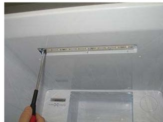
Same as disassemble of a freezer.
