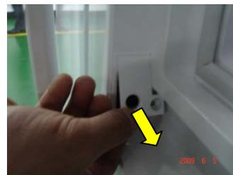
After loosen screw, pull and separate damper cover to arrow direction using a tool.
