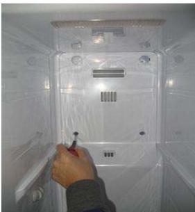
Separate fixing screw of a cooler fan cover.
