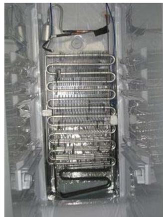
Figure of a freezer room after cooler front cover is removed.
