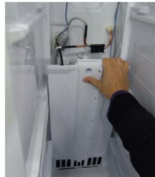
Separate the upper part of the Louver F B from the Freezer holding it and pulling it toward the front.
