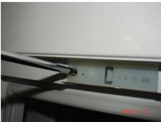
Remove the fixing bolt of the Ledge.
