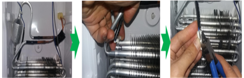
D-sensor disassemble
